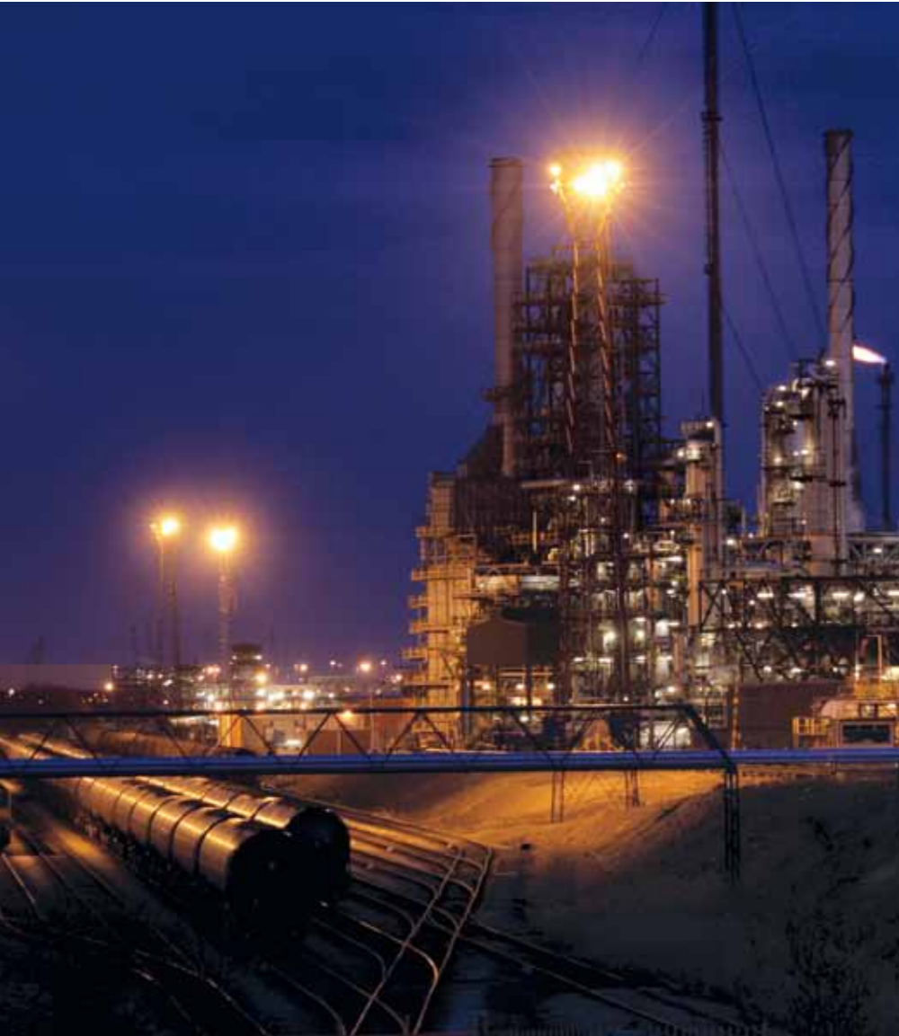
Total Lindsey Oil Refinery.
